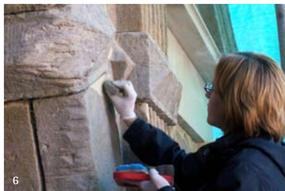
Above and right: Figs. 1-5 - Patching flaws with stone repair mortar Figs. 6/7 - Retouching repair work
