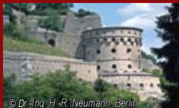
Machicoli Tower Würzburg / Germany
