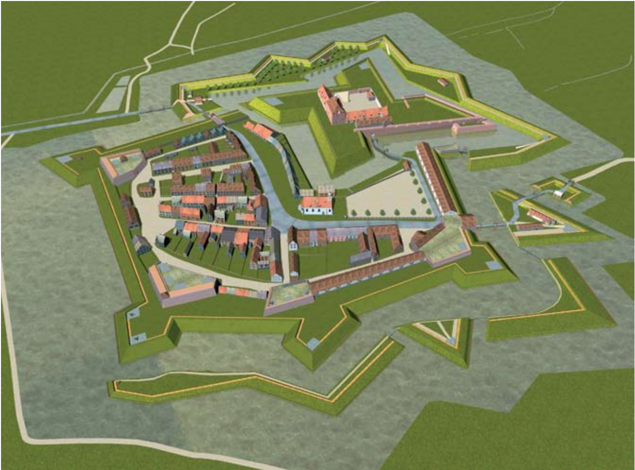
Fig. 4: Peitz. Digital isometric reconstruction of the fortifications around 1750 facing north. The sharply angled bastion at the centre front of the picture is the Malzhaus bastion. The Malzhaus bastion lay between the powder tower bastion (front left) and the Office bastion (front right). Today, only vestiges of the Malzhaus bastion remain.
