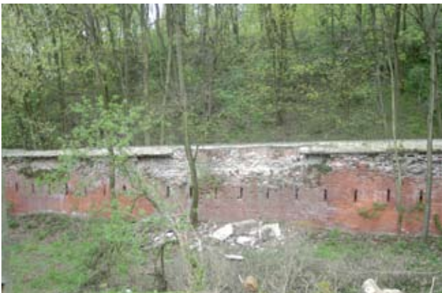
Fig. 60—62: Nowy Dwor Mazowiecki. Fortress Modlin. The structural maintenance of the works, such as the Carnot wall shown here within the citadel presents owners and operators with a tremendous challenge. The attack by nature is immense and continues to damage the brickwork.
