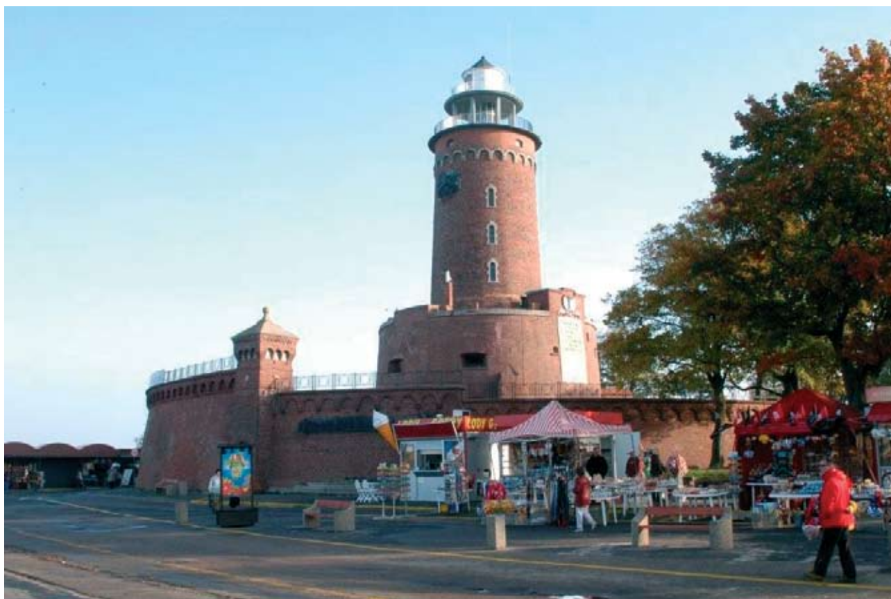
Fig. 10: Kolobrzeg. Fort Münde, present structure referred back to 1832—1836. The lighthouse was built on the fort in autumn 1945.
