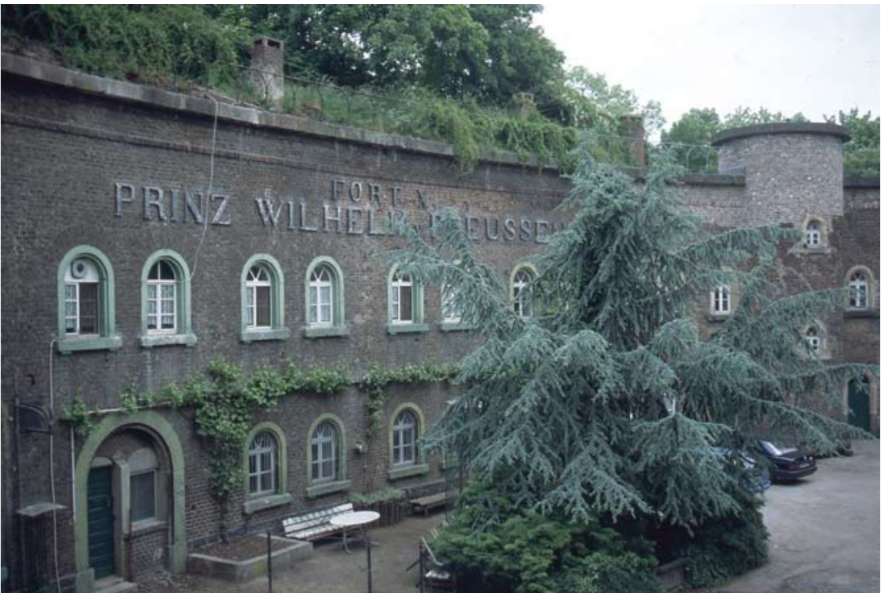
Fig. 101: Cologne. Fort X Prince William of Prussia on the left (Cologne) bank of the Rhine. The work is used by departments of the Cologne Garden Office. Status 1999.
