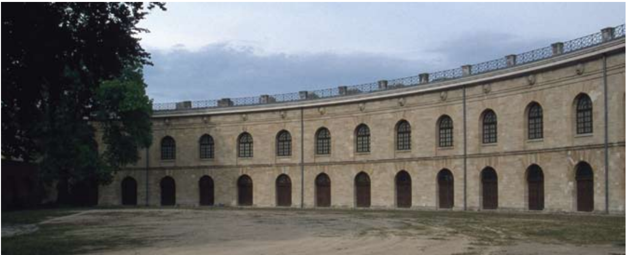
Fig. 141—144: Ingolstadt. Tilly Redoubt. Impressions from the bridgehead area. Tilly Redoubt: entrance gatehouse and frontage of the central structure. Above the cornice, the profile of the rampart as a stone finish. The access gate to the right and parade ground below.
