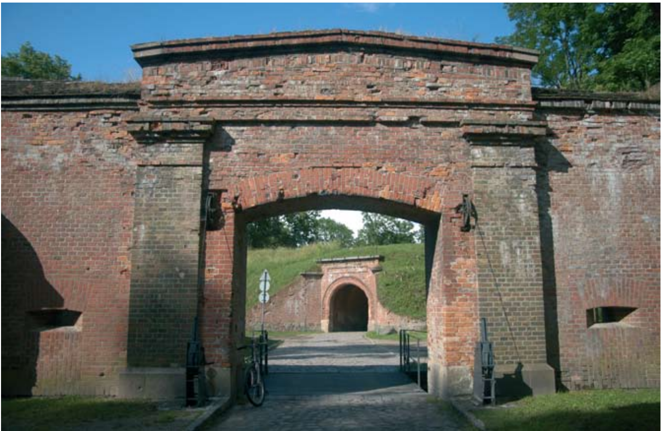
Fig. 20: Giżycko. Boyen fortified complex, view from the inner parade towards the main entrance gate.
