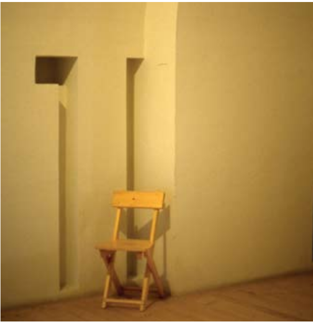
Fig. 145—146: Ingolstadt. Tilly Redoubt. During the plastering work, particular care was taken with technical details in the casemates, unlike the case at Fortress Ehrenbreitstein. Here, all the recesses for anchoring the wooden beams, which were to serve to safeguard the casemates and separate them from each other in wartime, are still existent.
