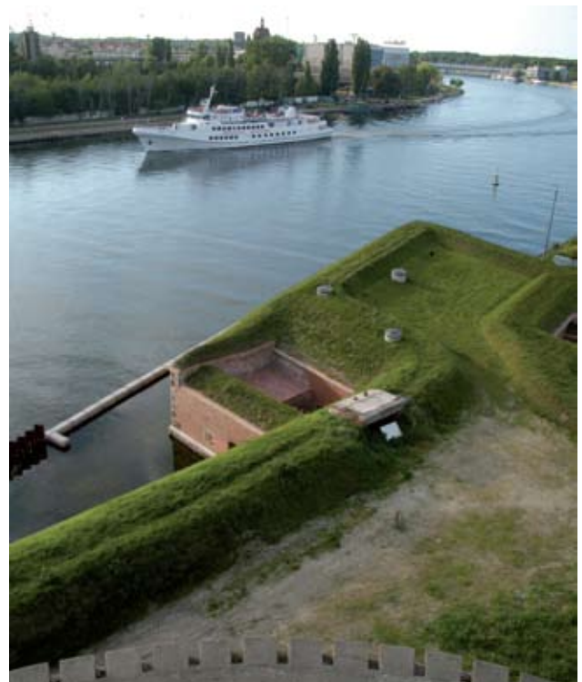
Fig. 57: Gdansk. Fortress Wislamouth. The mole in front of the bastion provides protection from the wakes of ships entering the Vistula.
