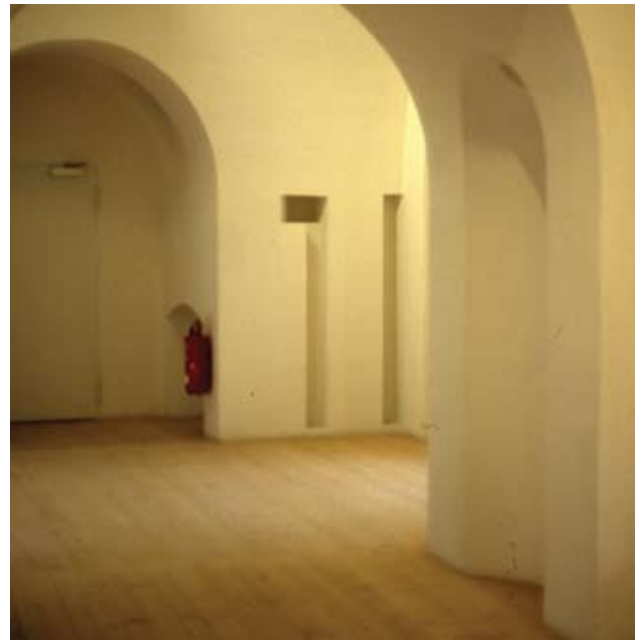
Fig. 145—146: Ingolstadt. Tilly Redoubt. During the plastering work, particular care was taken with technical details in the casemates, unlike the case at Fortress Ehrenbreitstein. Here, all the recesses for anchoring the wooden beams, which were to serve to safeguard the casemates and separate them from each other in wartime, are still existent.
